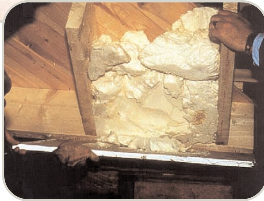
Images of UFFI above courtesy of Carson Dunlop. Copyright 2003, Carson, Dunlop & Associates Ltd.
